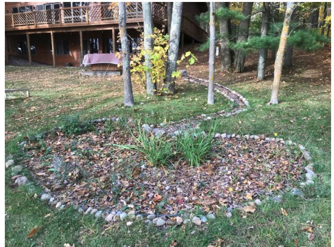
At Phil & Gretchen Takkunen's property, rainwater comes out of the downspouts, runs down the hill through drain tile, and feeds a rain garden with native plantings.
