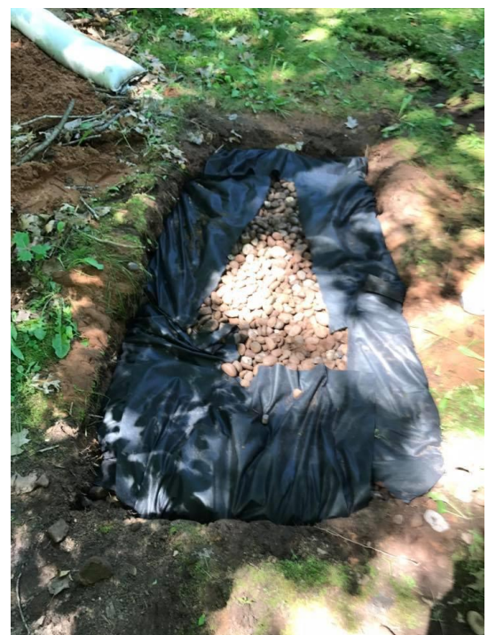
In-progress photos of one of my rock infiltration pit projects
